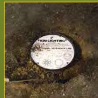
Secure debris shield cover and back fill soil.
