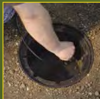
Attach intermediate connector to splice cover cap.
