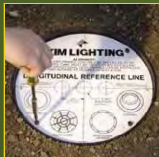
Remove debris shield cover.
