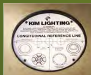
Pour Box with debris shield installed in concrete.
