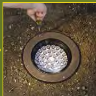
Attach component housing to molded housing.
