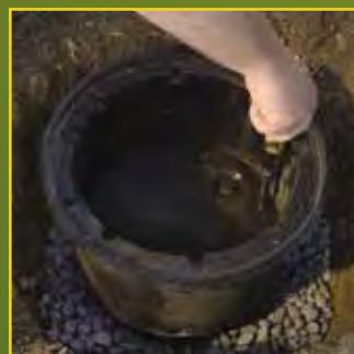
Place and secure splice cover.
