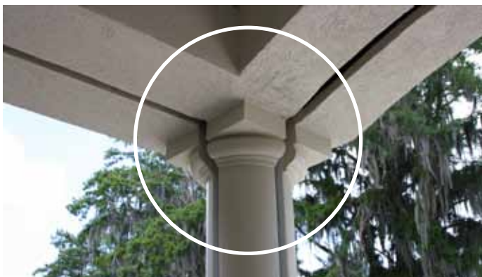
Recessed mount Executive screens showing screen opening and recessed U-channel built into fiberglass Roman columns.
