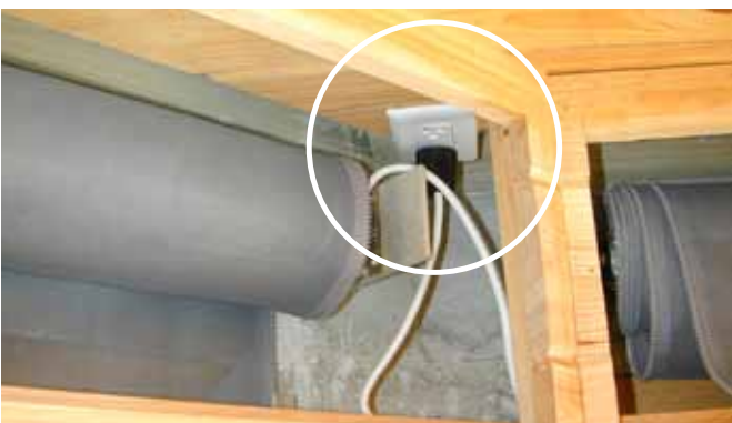
Duplex electrical outlet installed inside the cavity outside the working area of the screen roller, mesh and motor.
