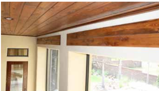
Removable front access panels finished to complement wooden tongue and groove ceiling.
