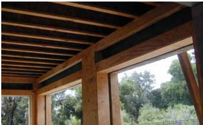
Cavity framed in top of header opening with front access. U-channel mounted in columns surrounded by framing before stucco finish is applied.
