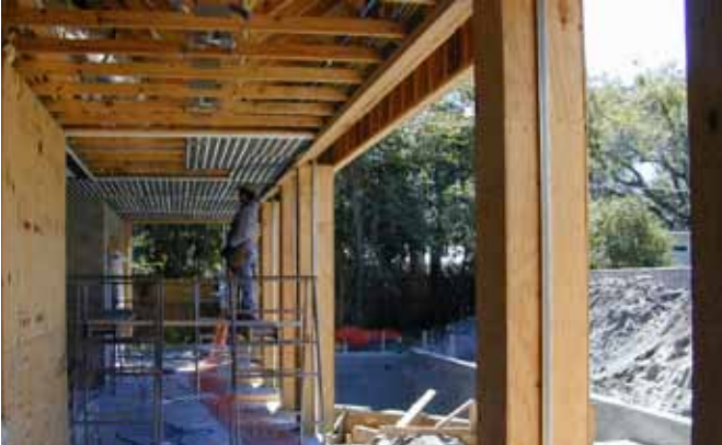
Cavity framed in top of opening with bottom access, u-channel mounted on column before finish is applied.
