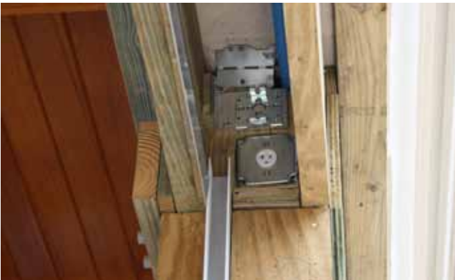
Unfinished cavity and column showing mounting brackets, electrical connections, and u-channel placement.
